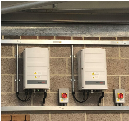
SolarEdge Inverter
