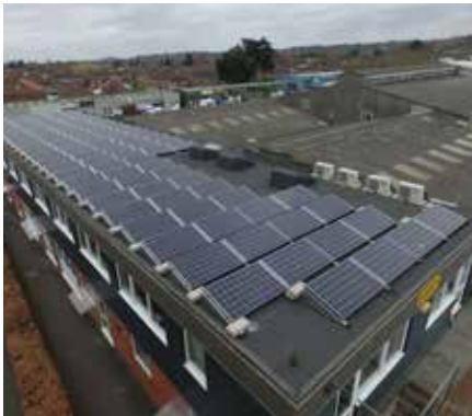
FLAT ROOF MOUNTING
