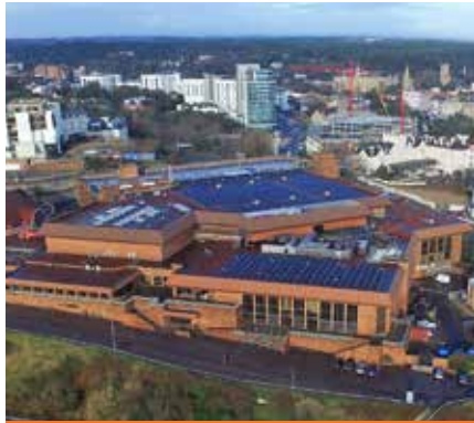
ARRAY - SUNEDISON PANELS
